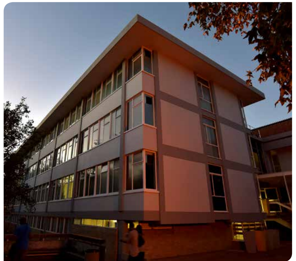
Office buildings, such as the Flippie Groenewoud Building, were upgraded.
