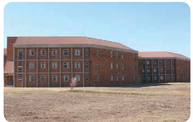
Steve Biko residence, seen from the west.
