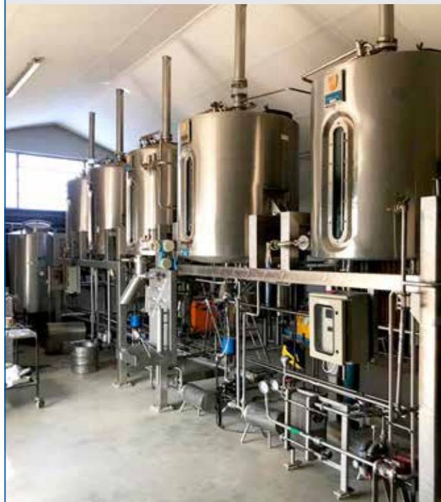
Current state of brewery installation
