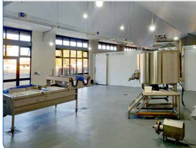
Dairy Processing Unit and the dairy processing equipment
