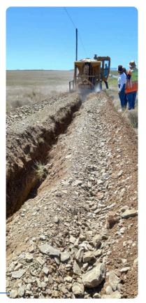
Excavating a trench in order to lay a fibre cable along the N8 route.
