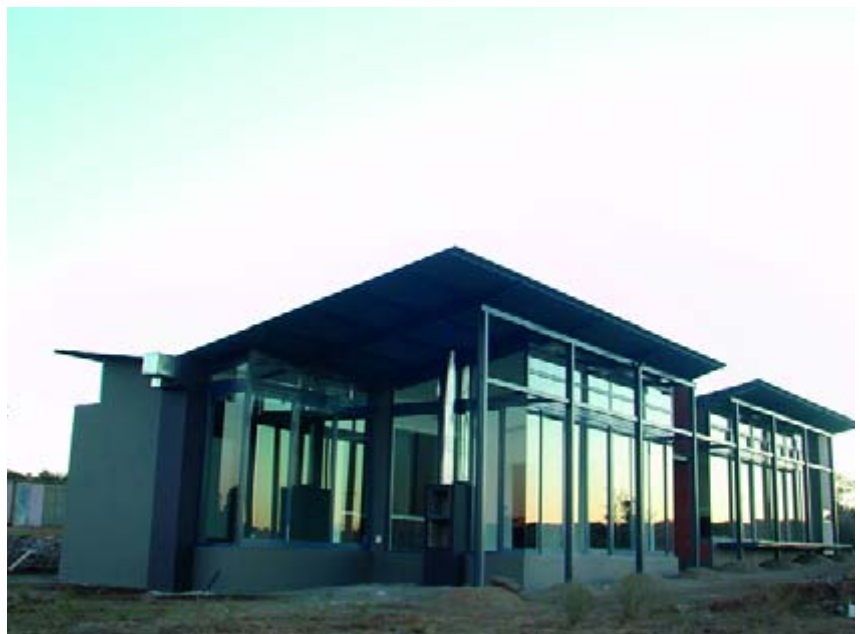
House Uys is situated in Rayton and was designed by Smt! Architects. It reflects farm architecture with its use of galvanised iron as building material.
