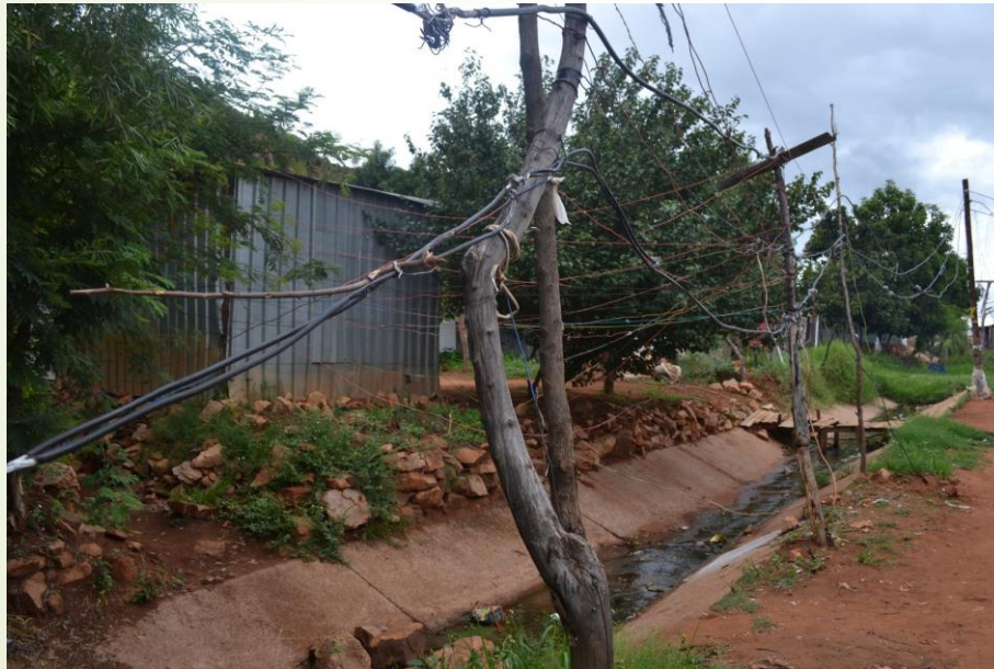
Illegal Electrical Connections
