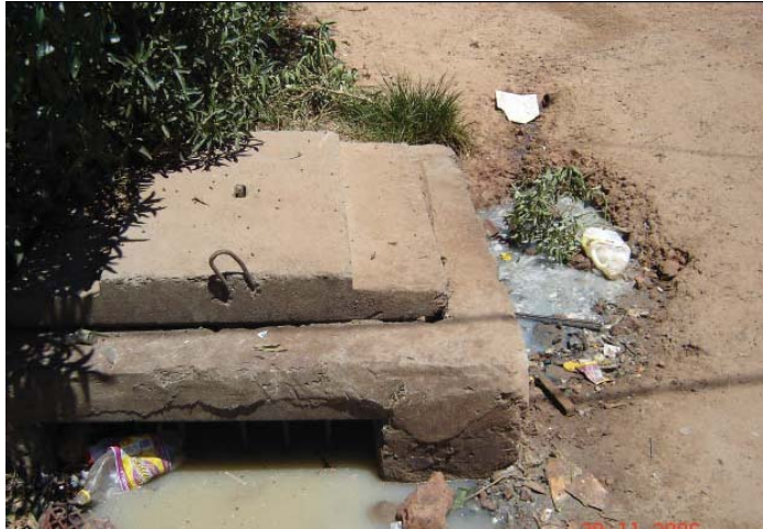
Figure 41: Blocked drains in Lusaka.
