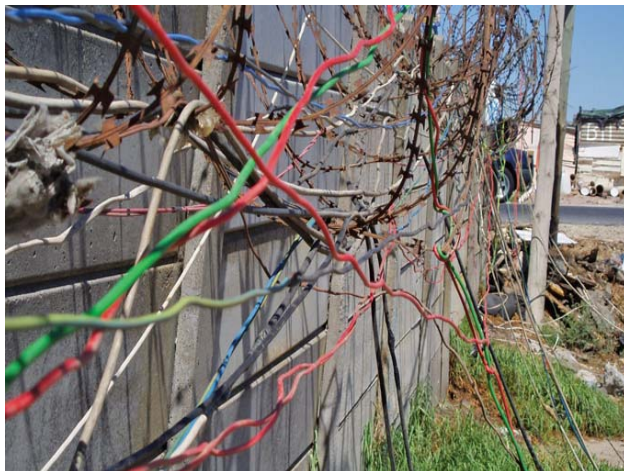
Figure 31: Illegal connection of electricity
