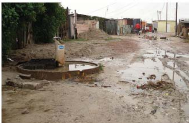
Figure 40: Accumulation of water around a poorly maintained community tap
