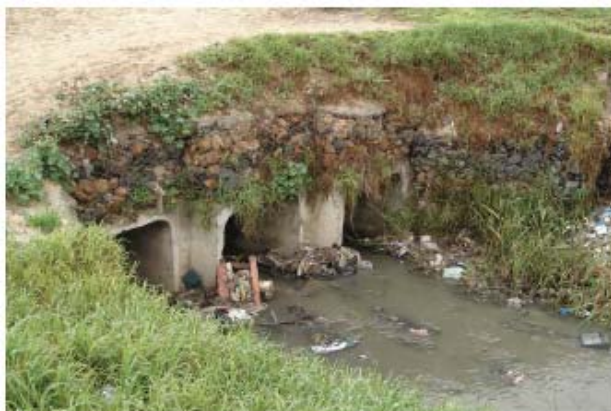
Figure 37: Drains clogged by waste on the stream Lusaka
