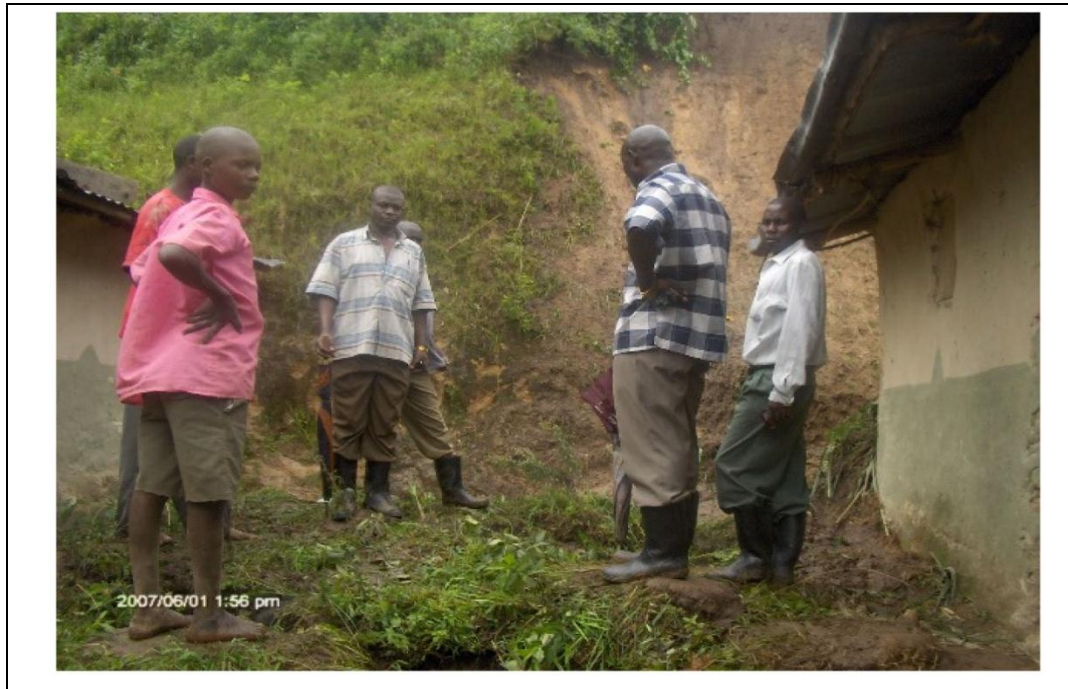
Figure 3: Landslide caused by undercutting of the slope for house construction
