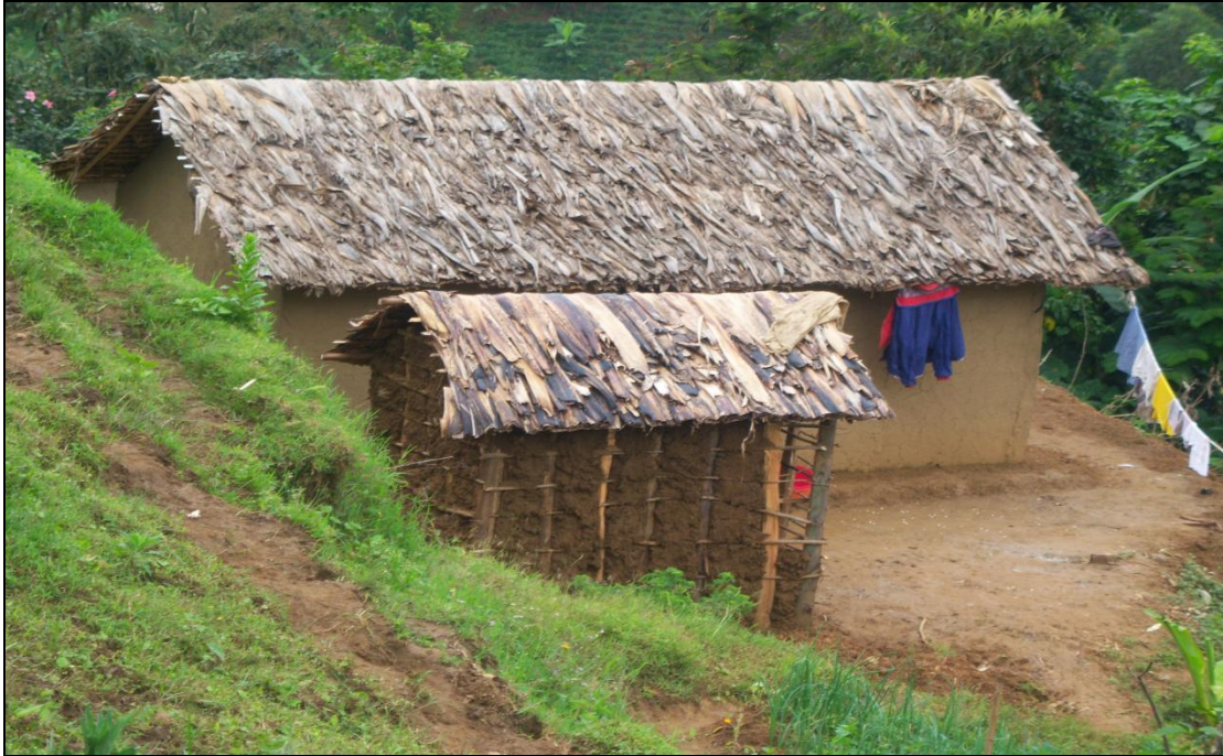
Figure 22: A kind of informal buildings in Bukalasi, Photograph taken during field study.
