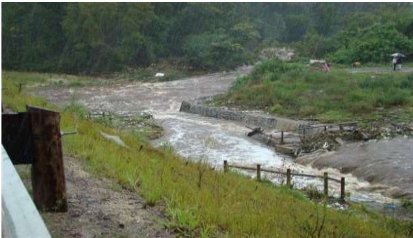
Photo 6: Storm water system filled with debris, near Thembaletu during the 2007 floods (George Herald, 2007)
