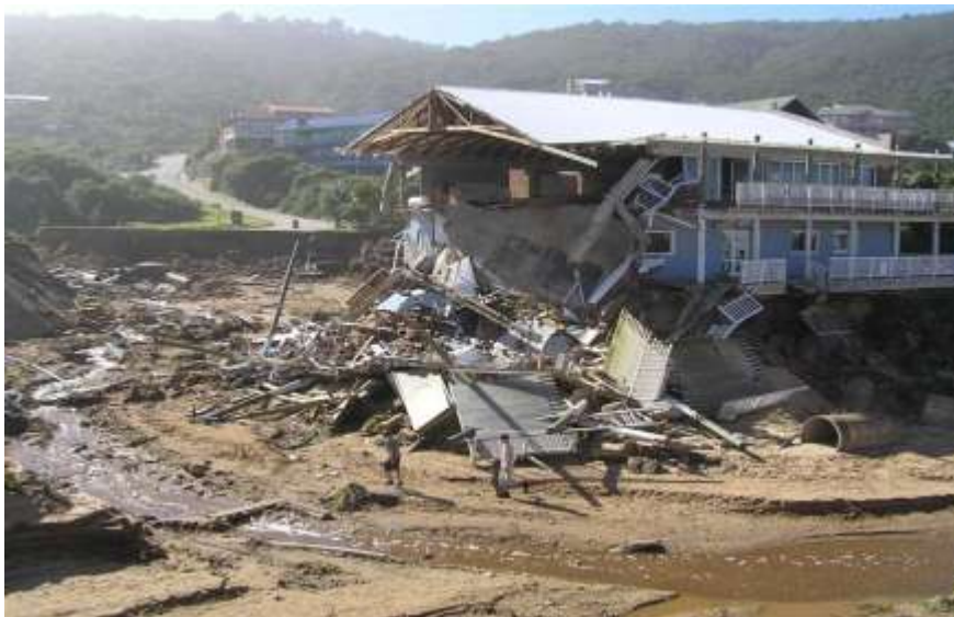
Photo 1: Photo of flood-damaged property in Glentana near Groot Brak River, after 2006 floods (George Herald, 2007)
