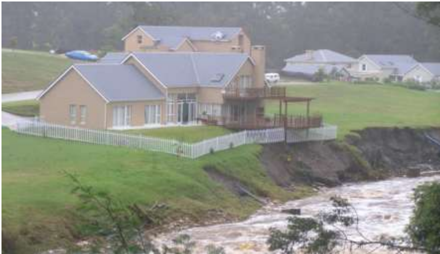
Photo 3: Property located on a low-lying area along a water course in Heather Park during 2007 after floods (George Herald, 2007)
