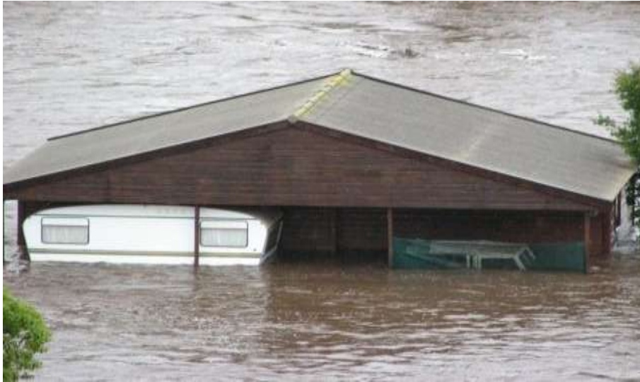
Photo 4: A wooden house build in a low-lying area near the Groot Brak River, which was immersed in water during the 2007 floods (George Herald, 2007).
