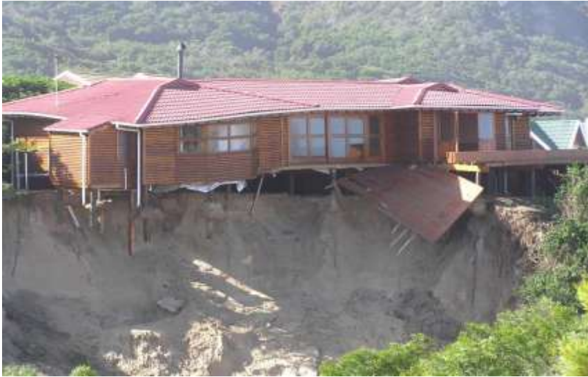
Photo 2: A flood-damaged house in Glentana constructed in a sand dune area during the 2006 floods near the Groot Brak River (George Herald, 2007)
