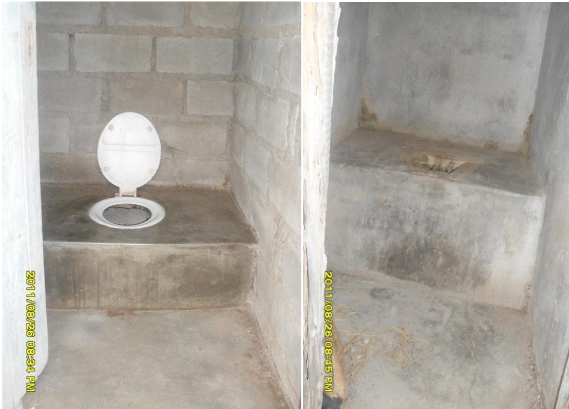
Illustration 12: Pit toilet with seat covers Illustration 13: Pit toilet without seat covers
