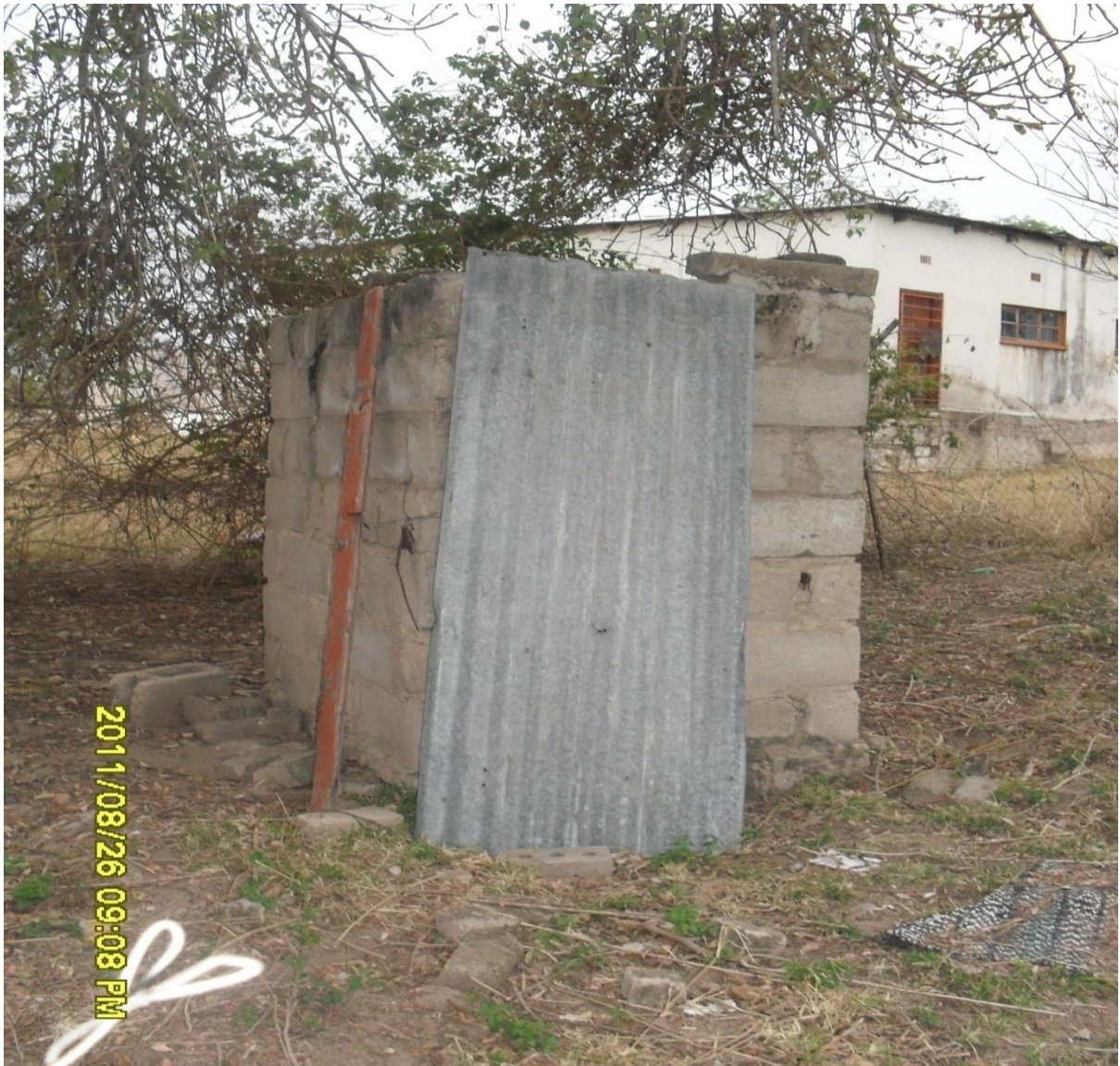
Illustration 10: the picture shows the poorly constructed pit latrine.
