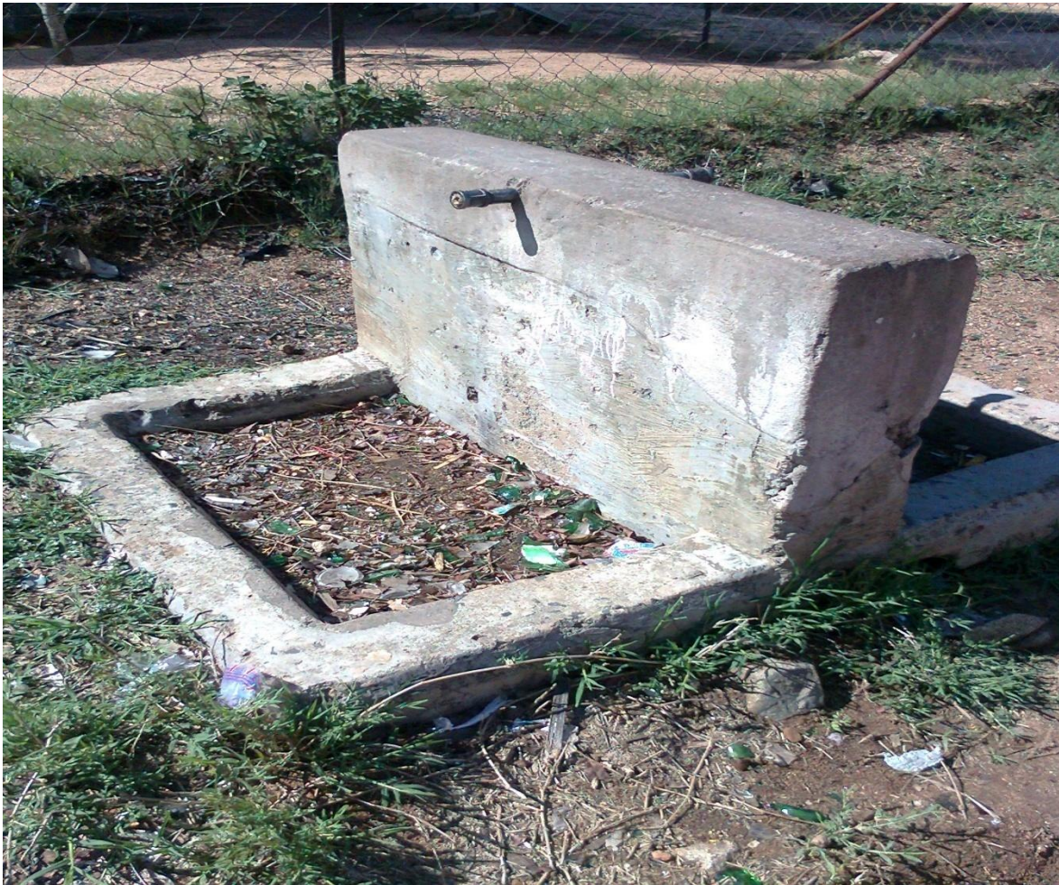
Illustration 5: An old village water tap that was no longer maintained
