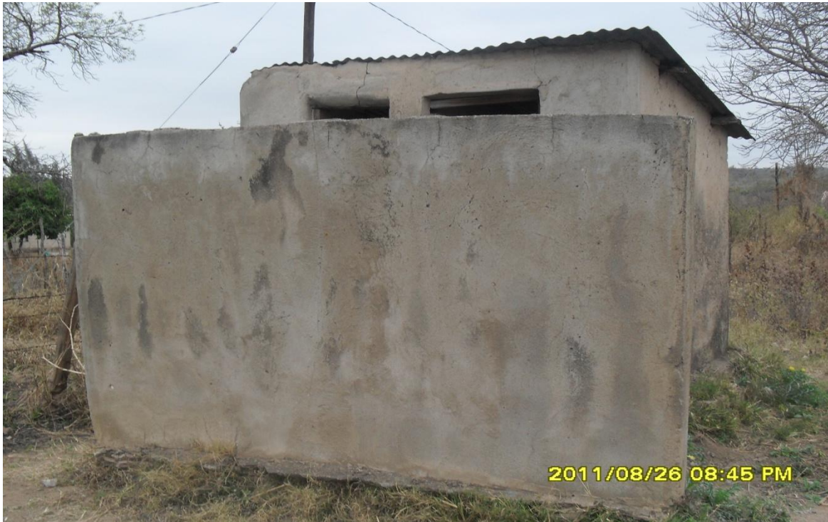
Illustration 11: Old double pit latrine
