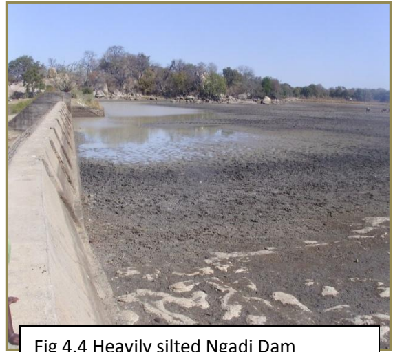
Fig 4.4 Heavily silted Ngadi Dam
