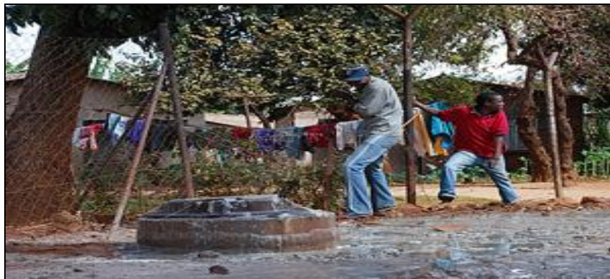
Figure 19: Youths trying to pass by a burst manhole in Old Magwegwe ( Source IRIN Africa 2008 )
