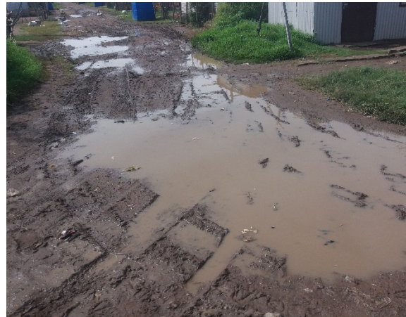
B. Example of bad roads and poor drainage systems
