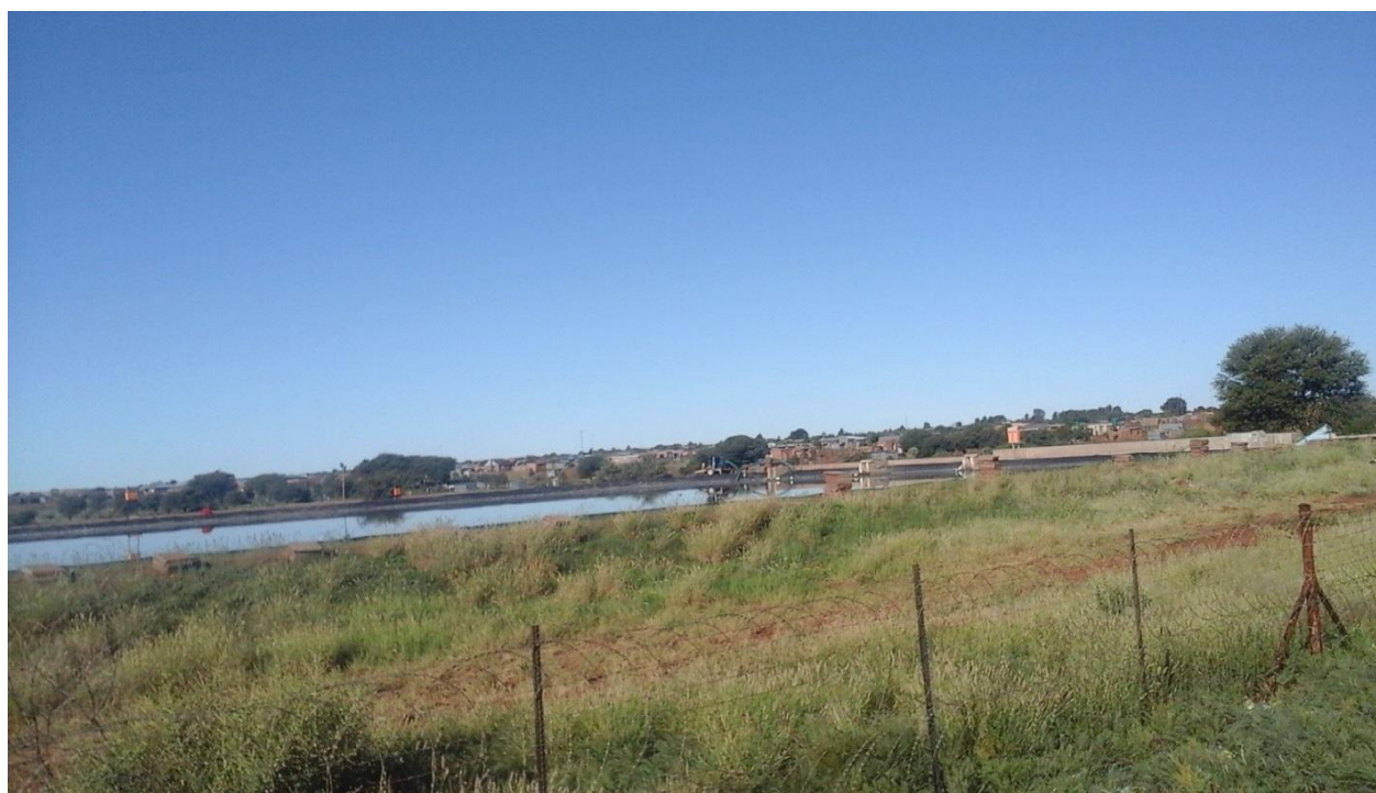
Figure 2.3: Sewage ponds serving sewage system of Mothibistad residential area
