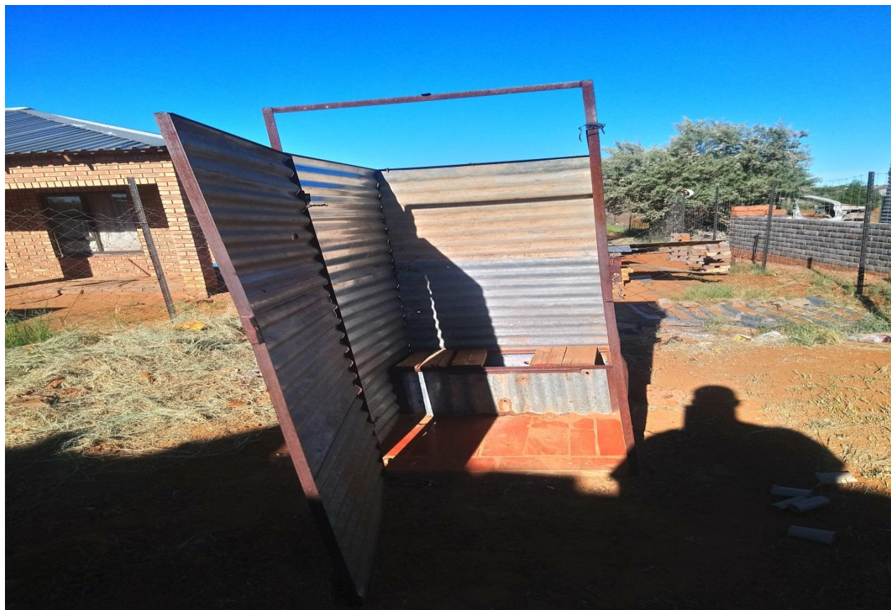
Figure 2 4: Pit latrine in Maruping village
