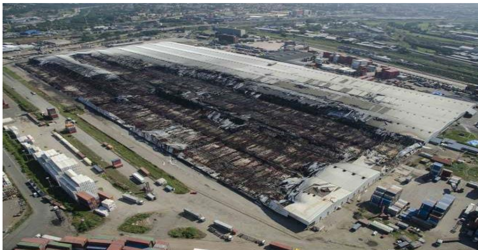
Figure 5.18: Warehouses that were affected after the fire Source: Transnet (2017)
