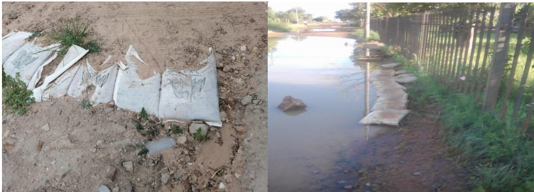
Figure 5.21: Shows sandbag flood mitigation measures implemented at Kudube informal settlement Source: Researcher
