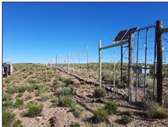
Klawervlei inspection site.
