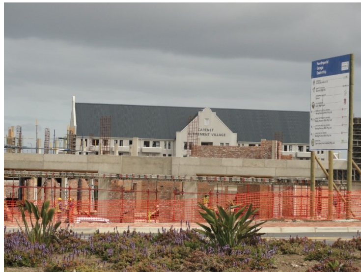
Photograph 11: Retirement development, 2013 (Photograph: Authors)
