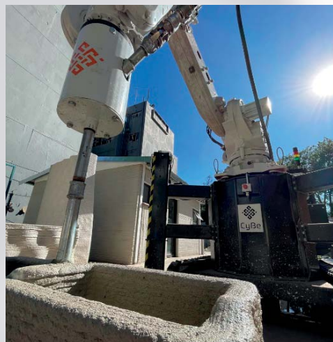
Figure 3 Researchers from UFS EnSci Green Concrete Lab are collaborating with University of Johannesburg on the formulation of 3D printable concrete mixtures based on agricultural waste
