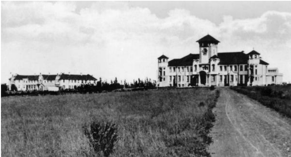
Figure 3: The newly completed Main Building and ManneteHuis (Later, in 1922, named, House Abraham Fischer) set in the Free State grass veld (FSPAR, Photograph no: VA 8132). 1909.
