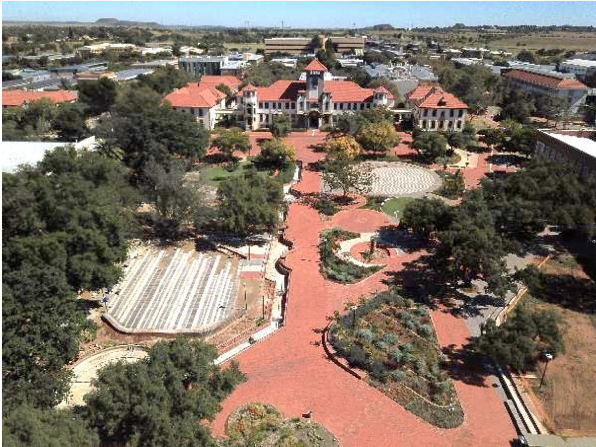
Drone photo of the Square, April 2021
