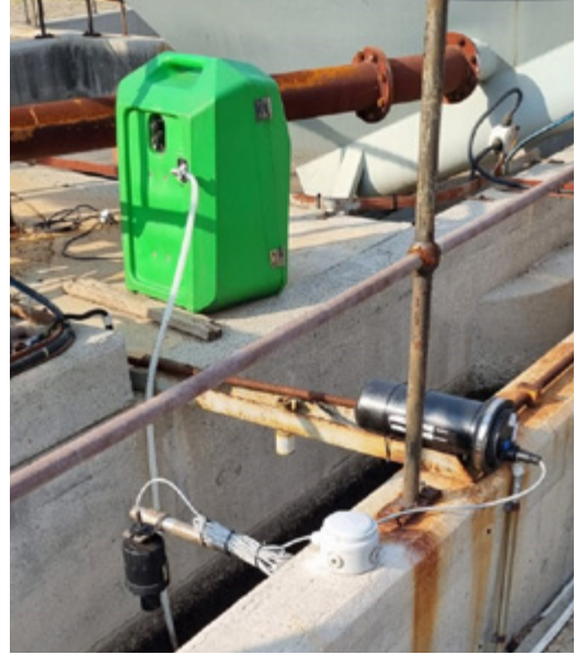
The flume at the WWTW with the sampler and secondary flowmeter.
