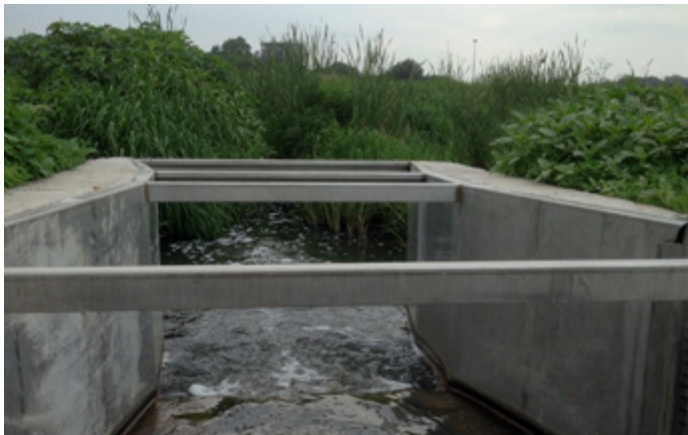
An engineered sluice enables wastewater velocity to be measured with great precision over a 24-hour period. This flow data, when correlated with viral load data, enables an accurate calculation of transmission dynamics in the population being serviced by a specific wastewater treatment plant.
